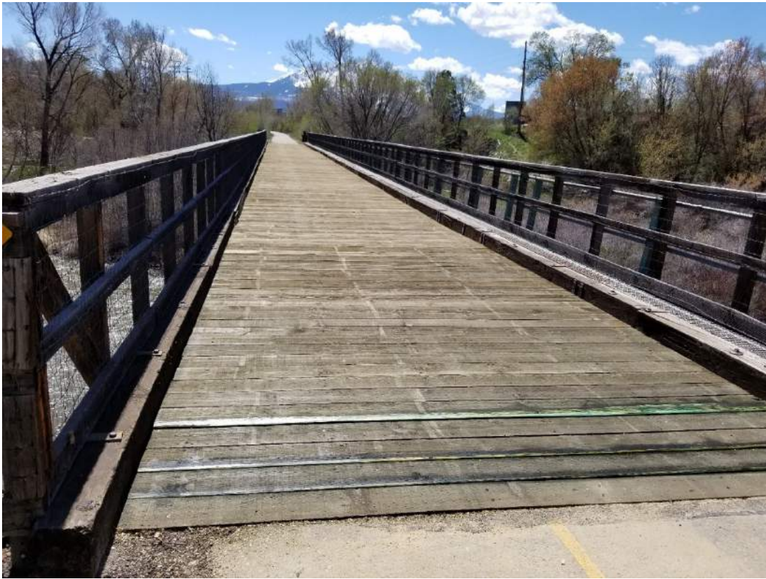
Roaring Fork River Railroad Trestle - Carbondale
