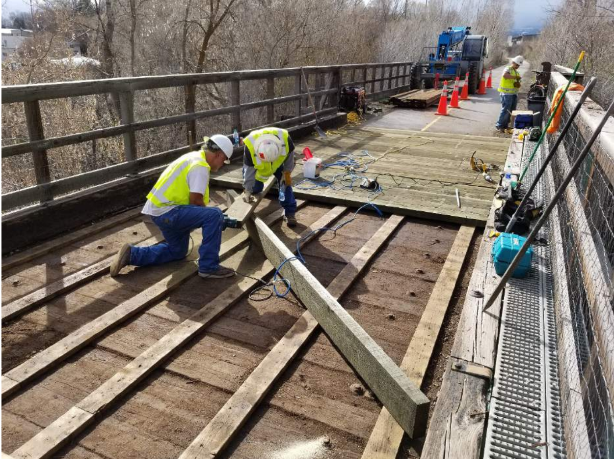
DECK RESURFACING ON THE ROARING FORK BRIDGE ON THE Rio Grande TRAIL
